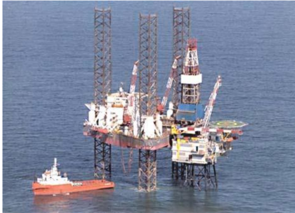
© Wintershall Q4-C platform, North Sea
