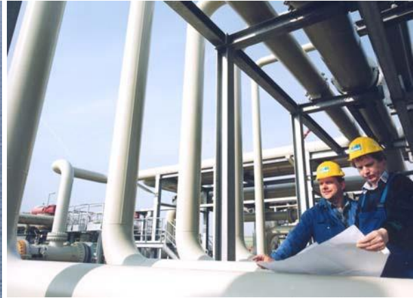
© Wintershall Wingas GmbH gasholder, Rehden (Germany)
